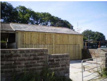
Notes: Slate roof. Block walls clad in timber.
