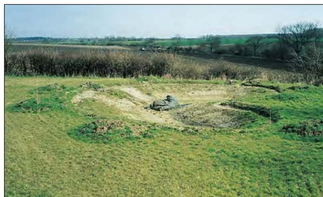
Lining a small (40m 2 ) pond on made-up ground. The pond has been dug and protective matting (centre) is unrolled to protect the underside of the heavy-duty butyl liner from below
