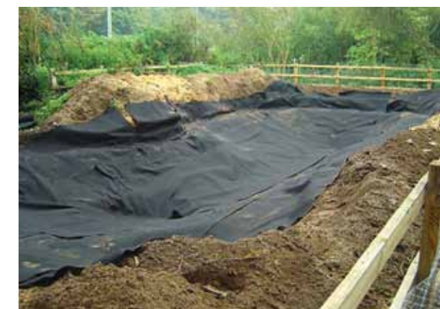
Butyl liner laid over geotextile underlay, Portal Woodlands, Ipswich. This liner required four people to lay (Duncan Sweeting)
