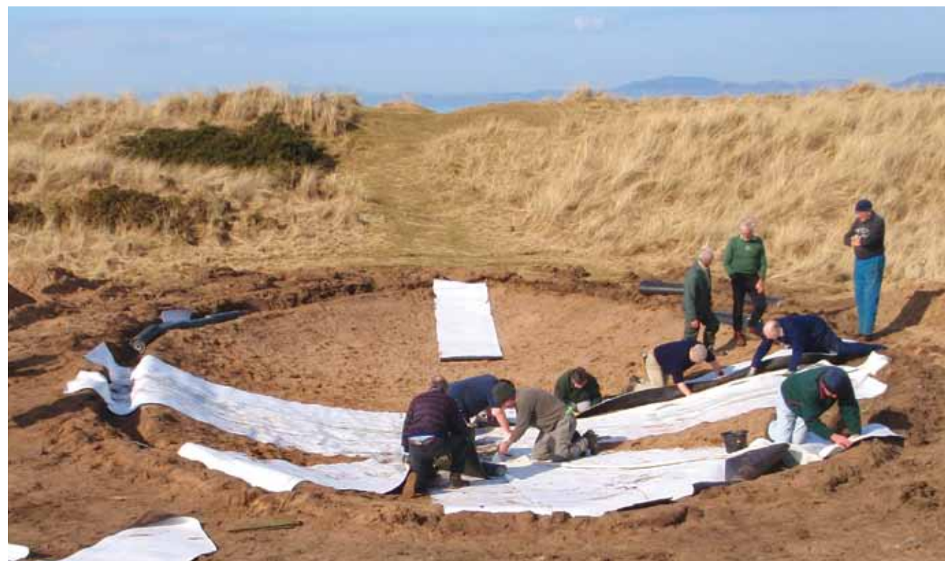
Natterjack scrape being lined with prehydrated bentonite (RAWMAT® HDB) at Mawbray Banks (Bill Shaw)
