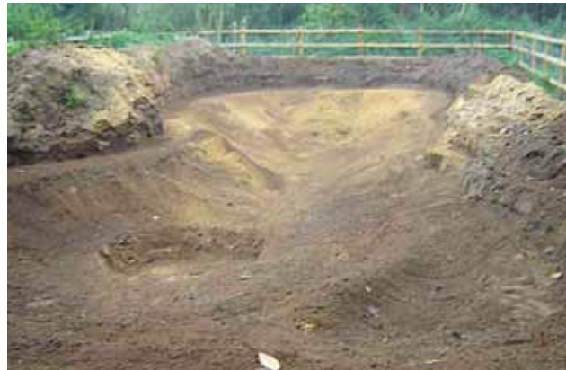
Here the butyl liner has been covered with a geotextile layer, topped with a 30 cm depth of sand from the excavation site (Duncan Sweeting)
