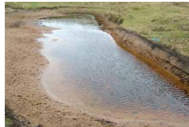
A scrape with an asymmetrical cross-section to give a shallow edge on the left and deeper water to the right (David Coward)
